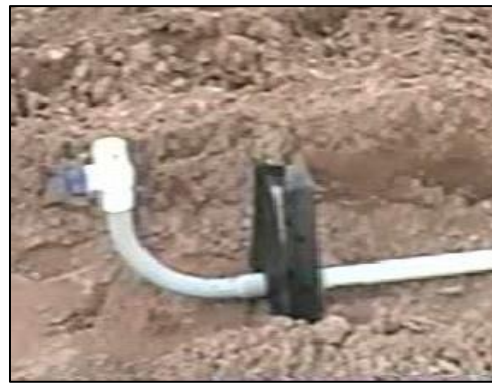
Figure 2: Sweep 90 with ball valve and end cap
